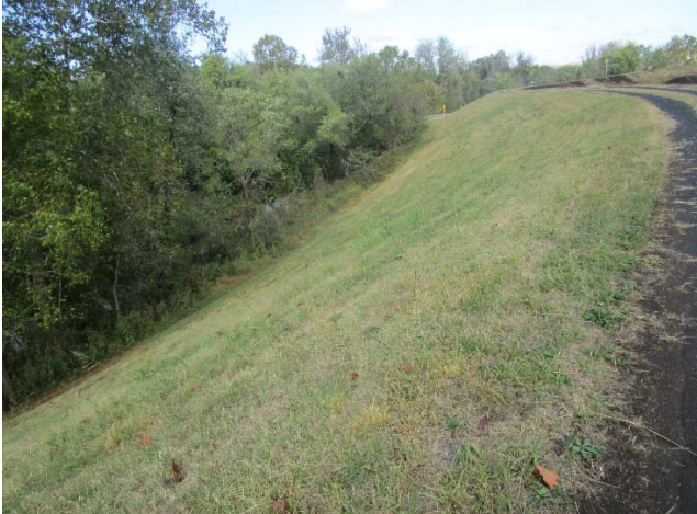
Photo 1 Typical view showing good conditions of the boiler slag embankment.
