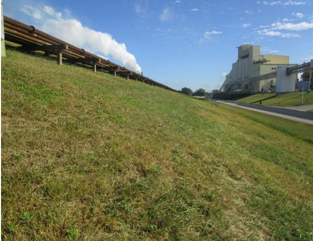
Photo 7 Typical view showing good conditions of the east embankment showing a uniform slope and a well maintained vegetative cover.
