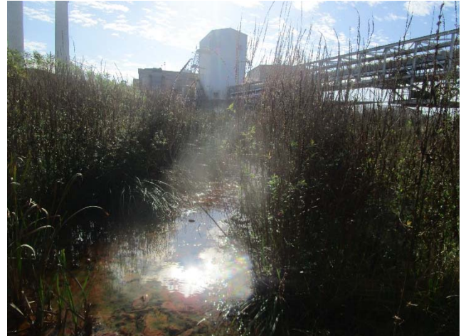
Photo 12 – Typical view of seep along the south dike showing a visually clear discharge.
