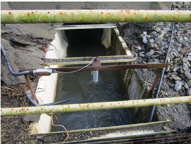
Photo 11 Typical view showing unobstructed flow from the south fly ash pond.
